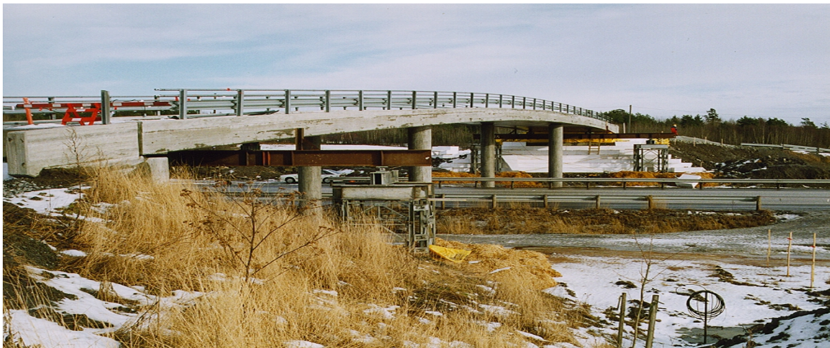
Figure 20. Temporary support of abutments at Hjelmungen
